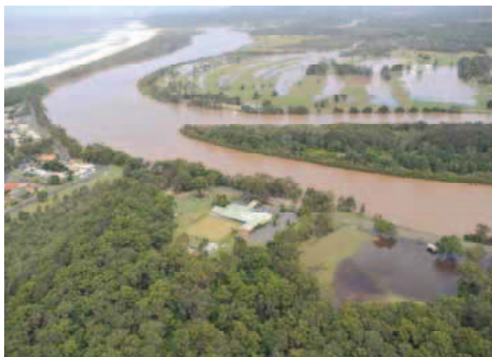
Figure 3.1. Bellingen River flooding at Mylestom (2009).
