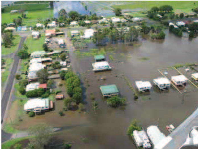
Figure 4.3. Flooding from the Richmond River at Coraki (January 2008).
